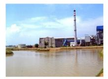
During 2009 at Unit 3, a massive pond covering an area of 7 acres was constructed to hold the rain water. The total volume of water that this pond can hold in each filling is about 56500 m<sup>3.</sup> Entire factory roof top rain water is being collected & channelized to this Harvesting Pond.
