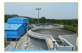
At Gingee, we have established a Water Treatment System in distillery plant, to treat the highly acidic condensate produced during processing of concentrated spent wash. This is treated through Anaerobic Digester and Extended Aeration Tank followed by Clarifier and is used for molasses dilution in Fermentation process.
